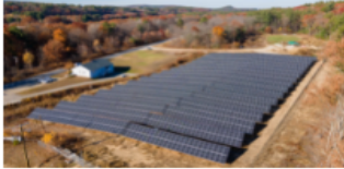
Hooksett Treatment Plant
